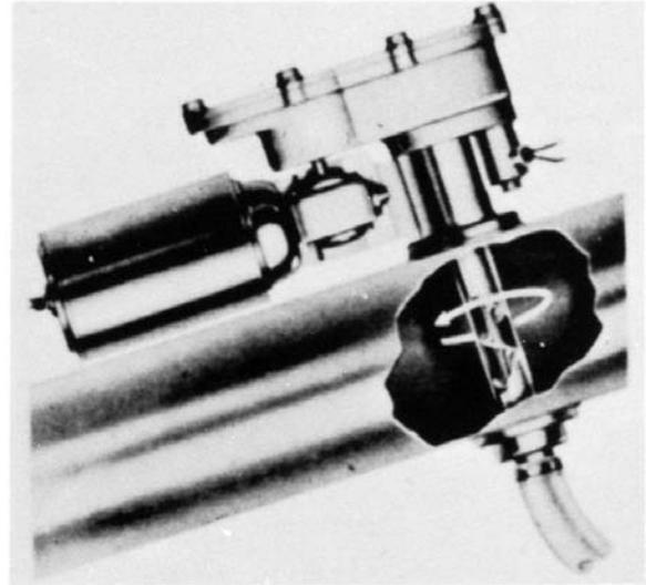
FIG. 16 Gravity-Flow Auger Sampler
